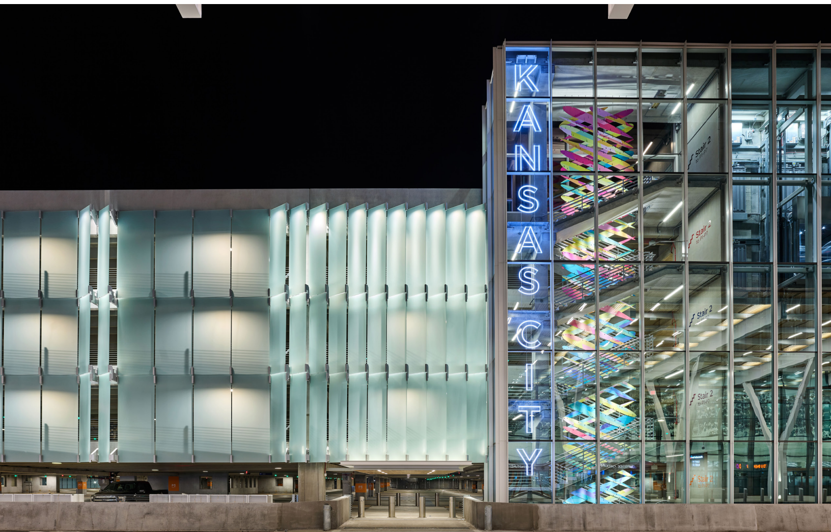
Kansas City International Airport New Terminal Parking Structure | Kansas City, MO
