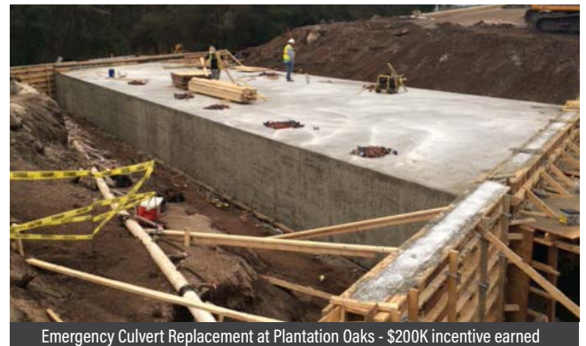
Emergency Culvert Replacement at Plantation Oaks - $200K incentive earned
