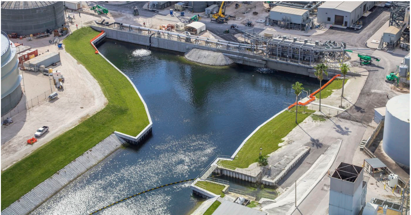
Florida Power & Light's Upgraded Port Everglades Power Plant, Fort Lauderdale, FL
