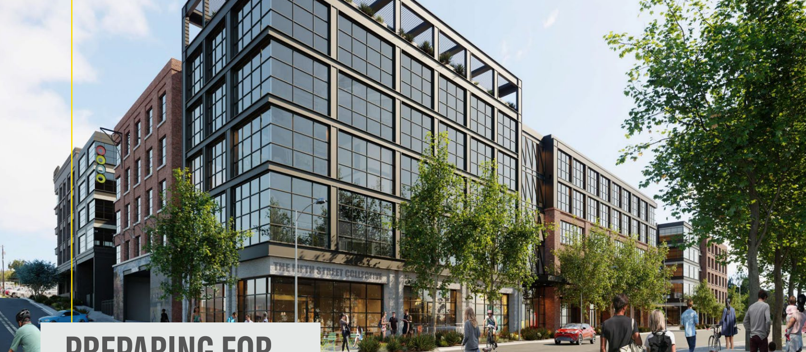
Centro West Mixed-Use Office Project, Austin, TX
