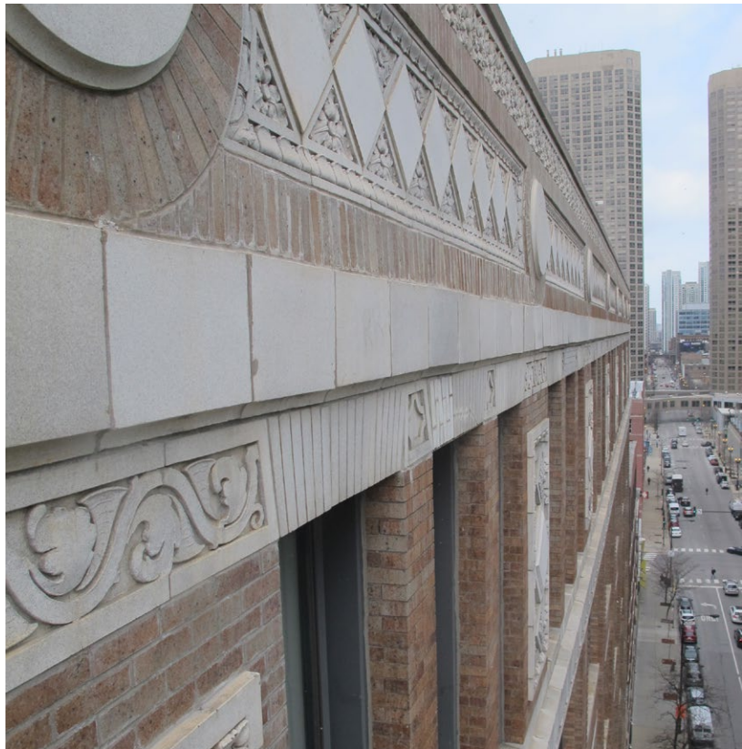
600 W Jackson Boulevard completed façade repairs
