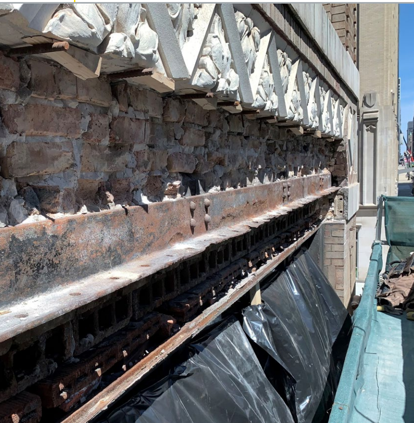
600 W Jackson Boulevard window lintels during façade repairs
