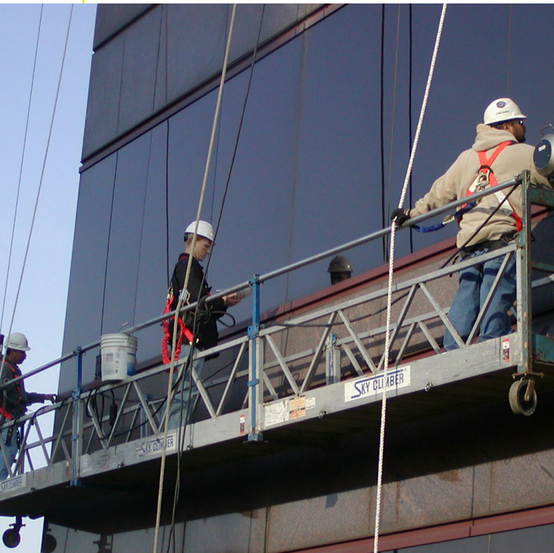
Curtainwall façade condition assessment
