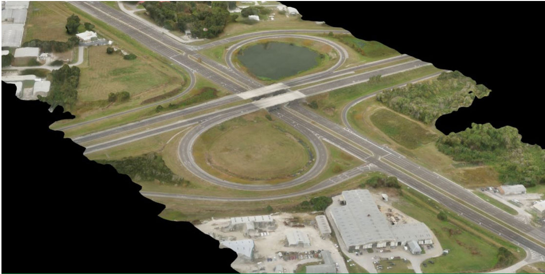
UAS Aerial LiDAR Scan of the Fort Frasier Trail Extension, Polk County, FL
